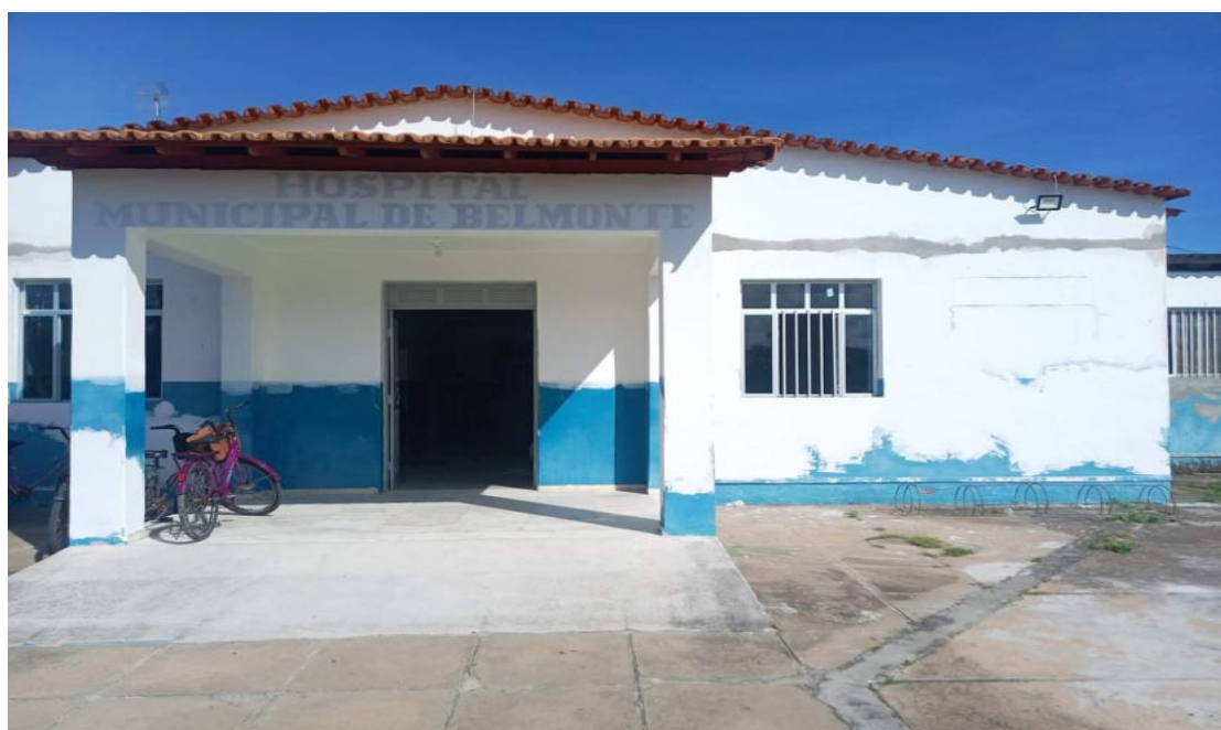
Hospital Municipal Durante a Reforma
