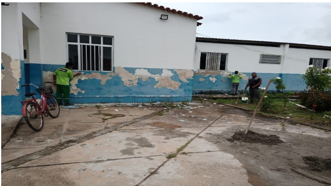
Hospital Municipal durante a reforma
